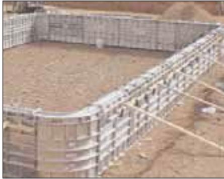
The Swim-crete system allows unskilled labor to be quickly trained in the use of the forming equipment. This is achieved by utilizing lightweight, high strength aluminum in the manufacture of the forms. This makes the modular system man portable and easy to assemble without the need of additional equipment.
