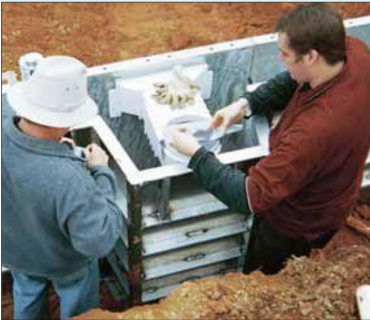
**Note: Always tape the top of the skimmer to prevent concrete leakage**
