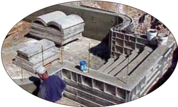
**Note: Remove all screws from forms where white goods are located prior to stripping forms.**
