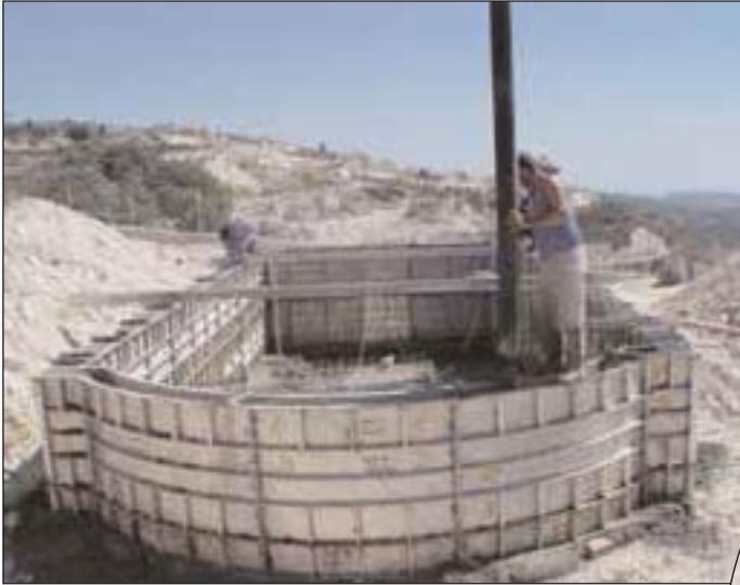
Concrete placement using the shear wall method achieves the monolithic concrete shell with a full depth vertical wall in the deep end.
