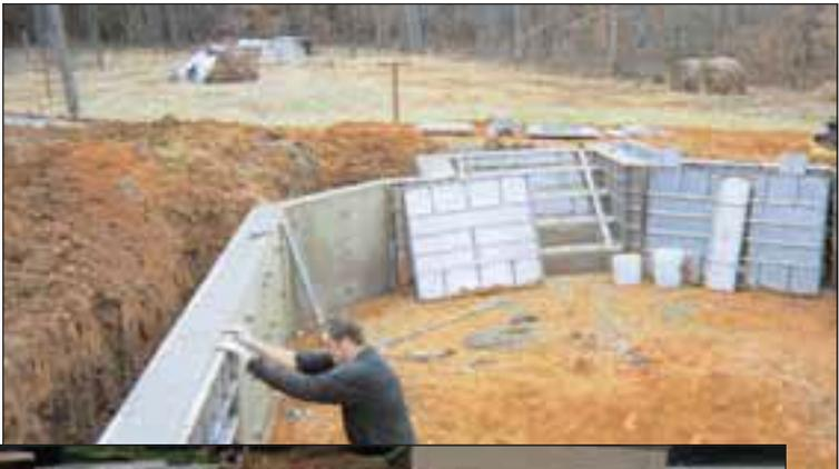
**The exposed tie ends are easily broken off using a standard hammer or the Swim-crete Tie Breaker Bar.**
