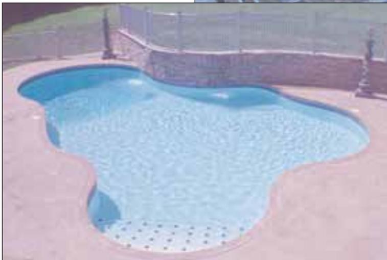
A retaining wall can be added simply by stacking forms and placing the concrete at the same time as the pool wall.
