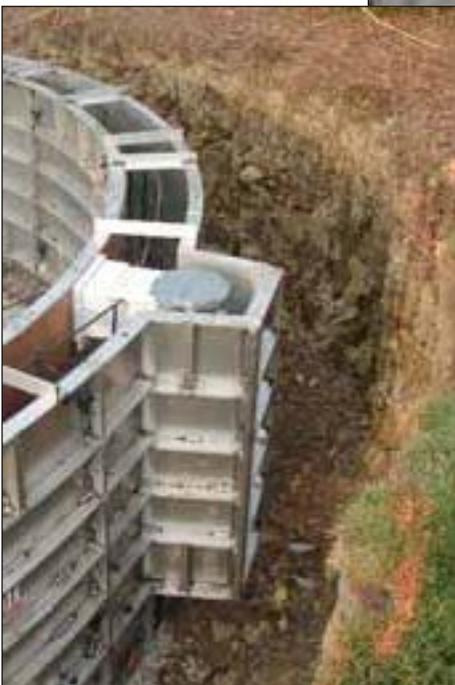
**3" (8 cm) slump recommended for all-concrete monolithic pool pours.**
